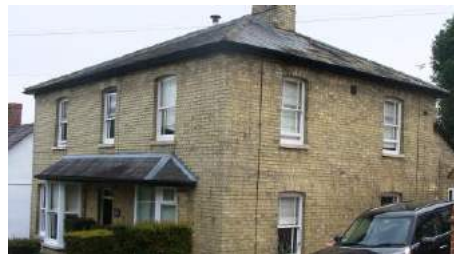
Picture 910 . Holly House a typical building of its type dating from the 19th century interpreted as having canopy to front added at a later date.
