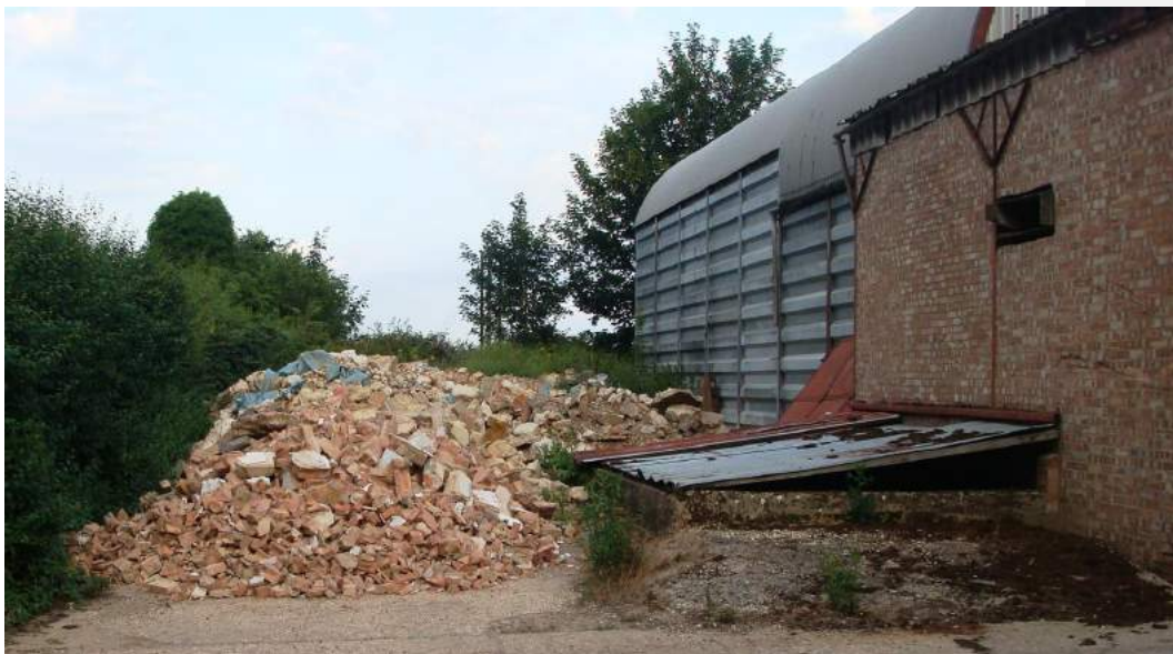
Picture 234. Brick rubble adjacent to the conservation area detracts. Hopefully discussions with the owner may secure improvements.
