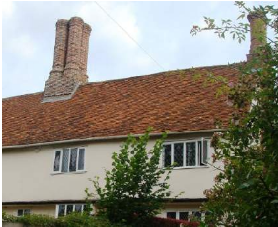
Picture 42. Fine chimney detailing, The Old Rectory.
