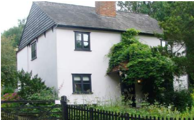
Picture 78. Swords Close a simple building of 19th century date that adds to the historic and architectural diversity of the street scene.
